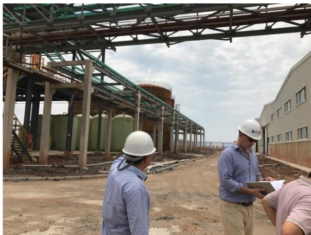
FIGURE 3: PLYMOUTH STAFF INSPECTING EXPANSION CONSTRUCTION ON A LITHIUM MICA PLANT IN CHINA
