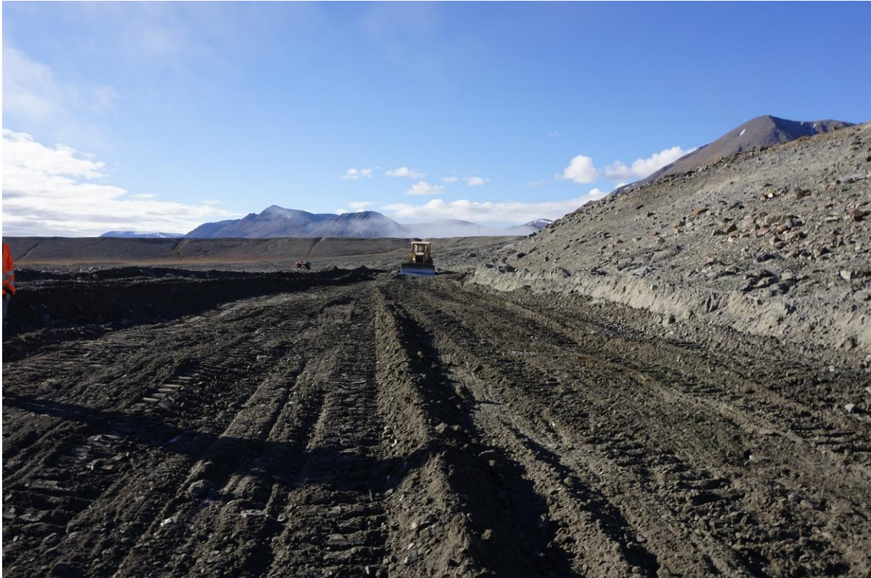
Figure 3: First cut of footprint to the porthole
